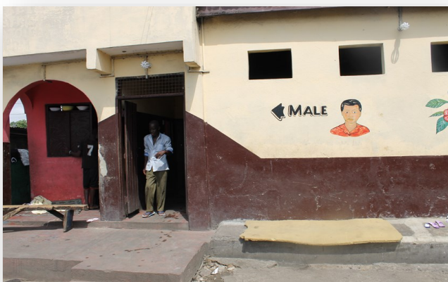
Figure 1: Man exiting public toilet in Accra, Ghana.
